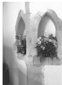
The piscina, which would have had the altar to Our Lady beside it.
